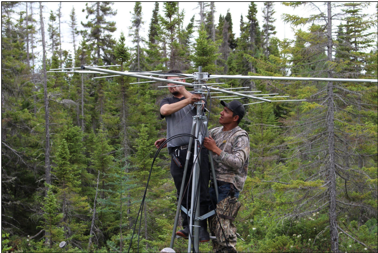
Figure 9: EMR-CTA staff installing the Motus tower in Boatswain Bay.
